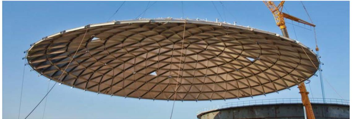
The HMT Aluminum Dome is a clear-span, lightweight, corrosion-resistant structure that sets the standard for performance in aluminum domes. The design complies with the latest edition of API 650 Annex G and the Aluminum Design Manual.
